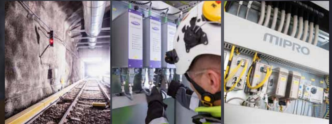
Mipro's metro interlocking system is based on object-oriented design and programming principles and thus provides centralised, distributed or mixed architecture solutions for various environments, depending on the customer's requirements. The distance between interlocking and field elements and the cable-laying work can thus be optimised and minimised.
