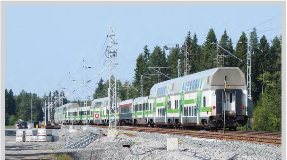
Figure 2: In the Kokkola–Ylivieska double track project, the continuously running train traffic sets the preconditions for construction work.
